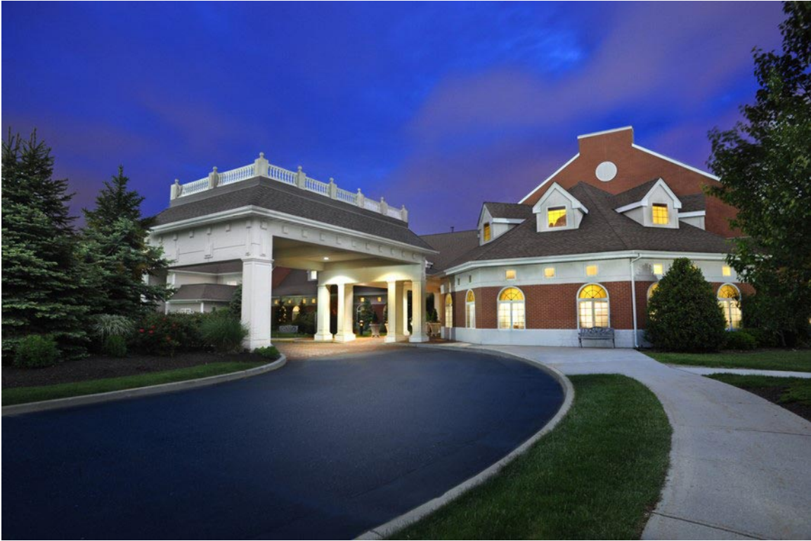
Jefferson's Ferry – Community Center Entrance
